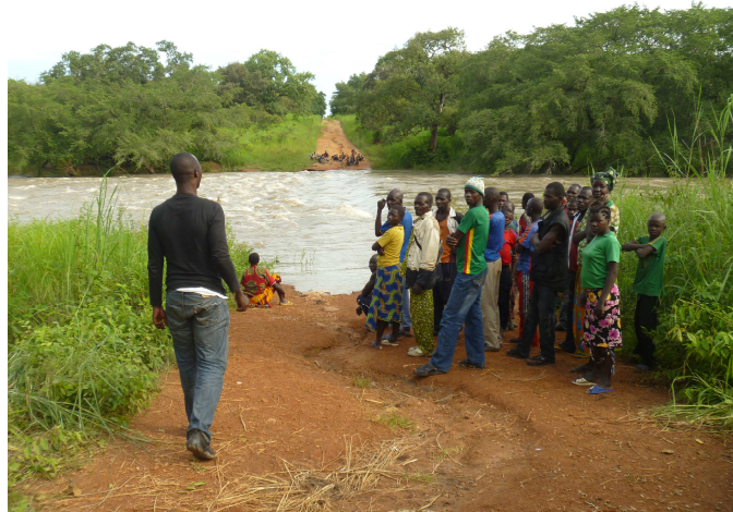
Figure 1 Road to Kaga-Bandoro cut-off by rains
